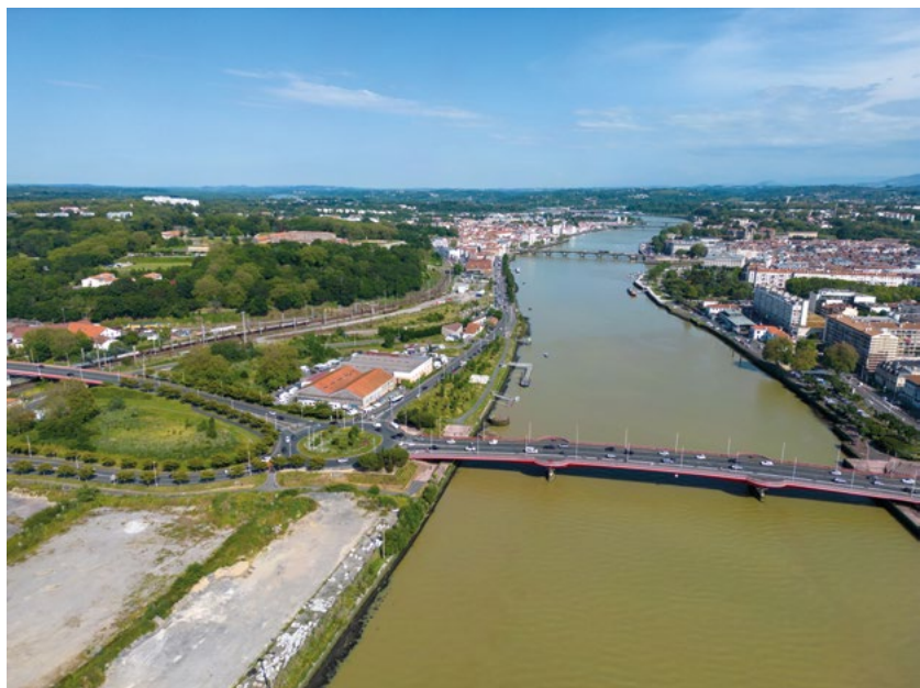
© Cote Sud Photo
